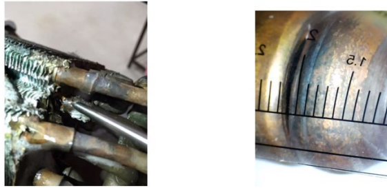
Figure 2: Holes in brazed fitting Source: Life Front – Recommended leak hole size and mass flow rates by system and application characteristics
